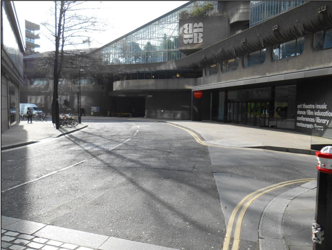
Barbican Centre entrance – before
